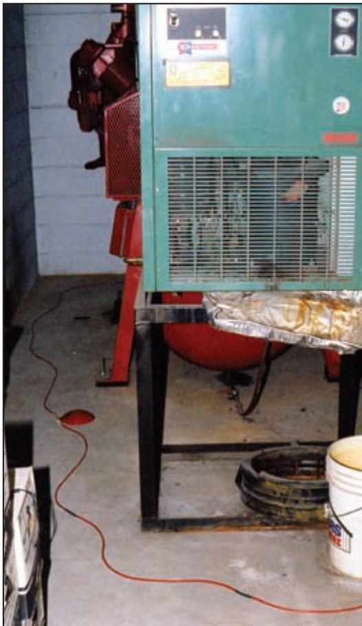
Water Alert / Sensor Cable in mechanical Room
